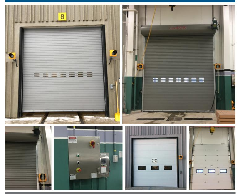
Address: North York, ON Contractor: Bondfield Management Inc. Equipment Provided: Cookson Model ESD-20 Insulated Rolling Steel Door Micannan PRO-GH Gearhead Operator
