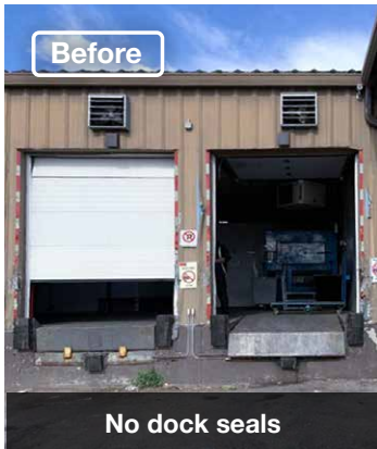
Gaps around trailers and damage to building
